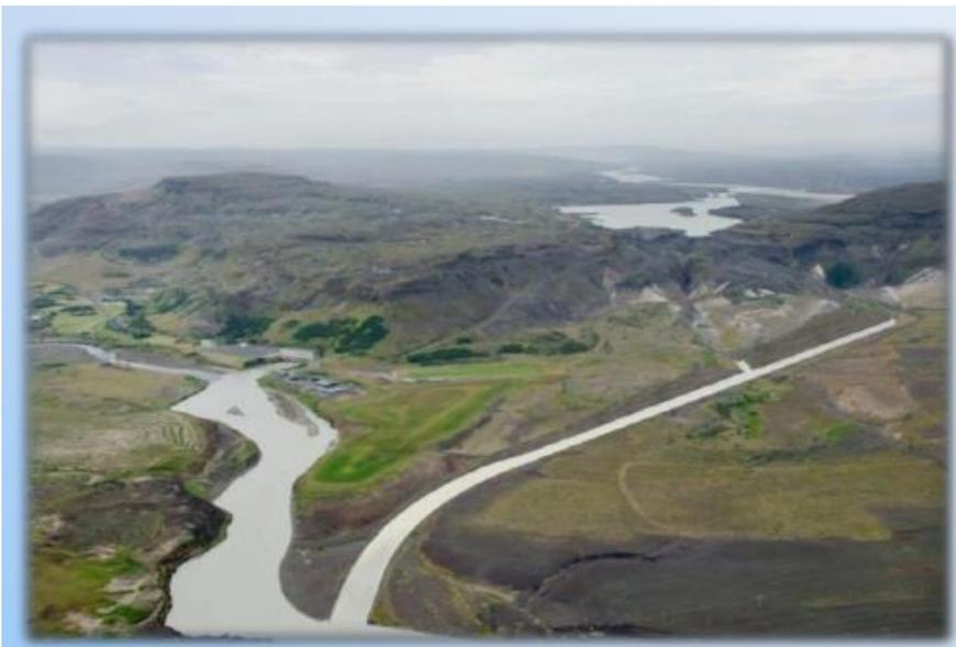
The construction of "Búrfell Extension HEP" was commenced in spring 2016, commissioning is scheduled for late April 2018. As the existing 270 MW power station, the new power station will be operated by water from Bjarnalón reservoir and have a capacity of 100 MW, generated by one single turbine.
